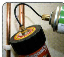
Our unique one way valve makes chemical dosing simple
